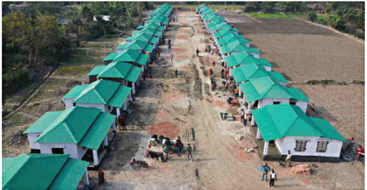
Houses for homeless at Gava village in Satkhira Sadar upazila.
