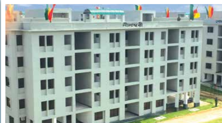
Constructed Building for Climate Victim
