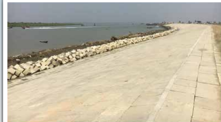
Protection Embankment beside Bakkhali River
